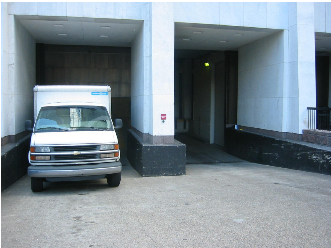
2 PHOTO AT ENTRY RAMP
