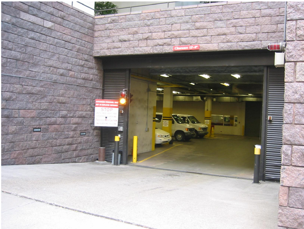
2 PHOTO AT ENTRY RAMP
